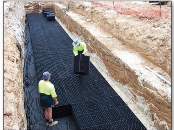
Installing the tank modules.
