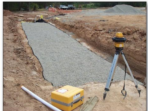
The completed tank covered with free draining material.
