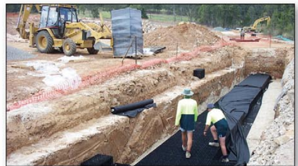
Wrapping the tank in Geotextile.
